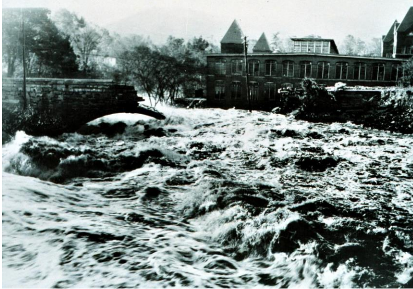
Flooding in Ware, Massachusetts effortlessly tore out a stone bridge. CREDIT NATIONAL WEATHER SERVICE
