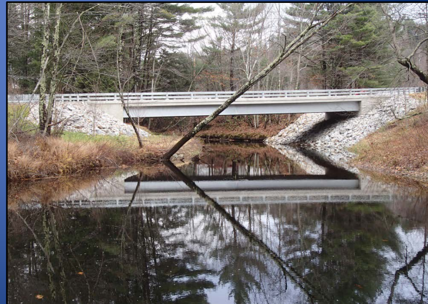
New bridge (80' span)
