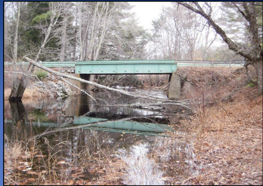
Pre-existing bridge (33' span)
