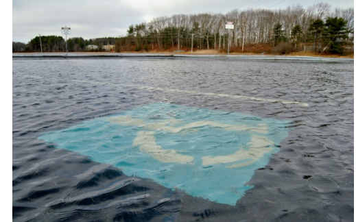
Low Lying Infrastructure
