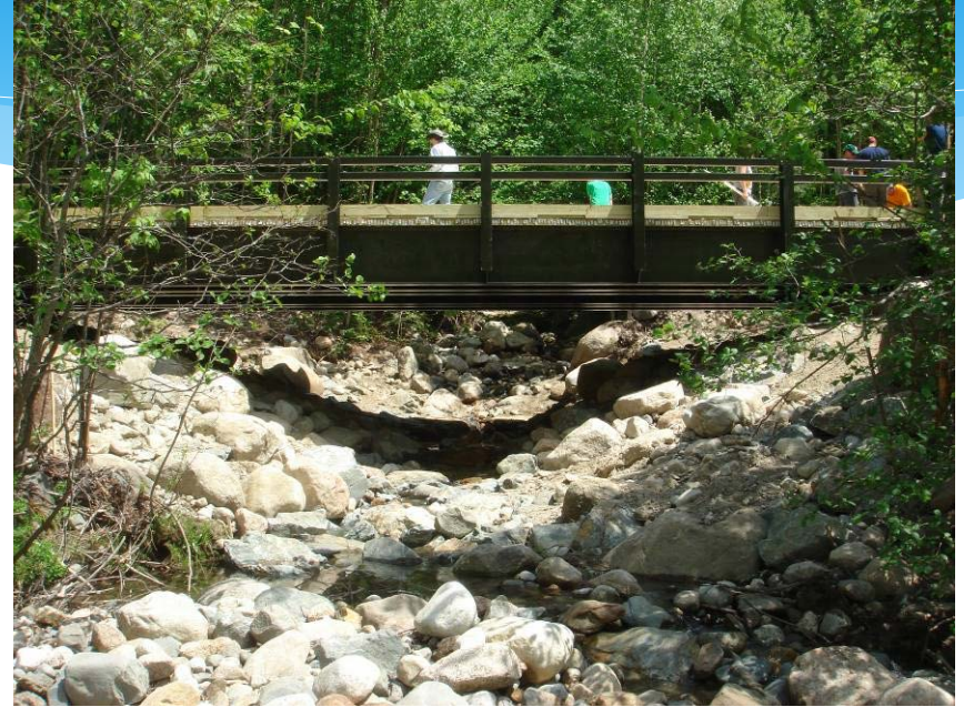
Post-replacement – looking upstream ~ 2010
