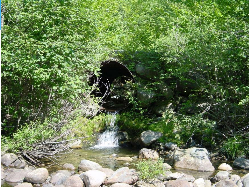
Pre-replacement – looking upstream ~ 2006
